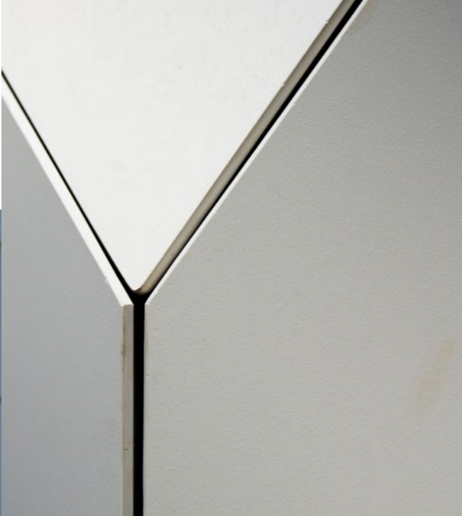
Fachada Eagle, Brisbane. Australia
